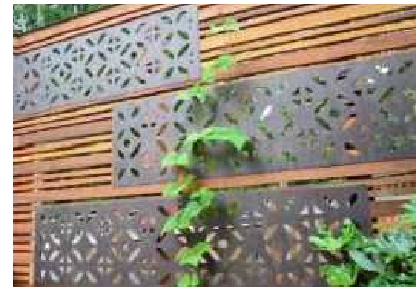
RAILING REFERENCE IMAGE
